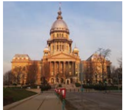
Illinois State Capitol building
